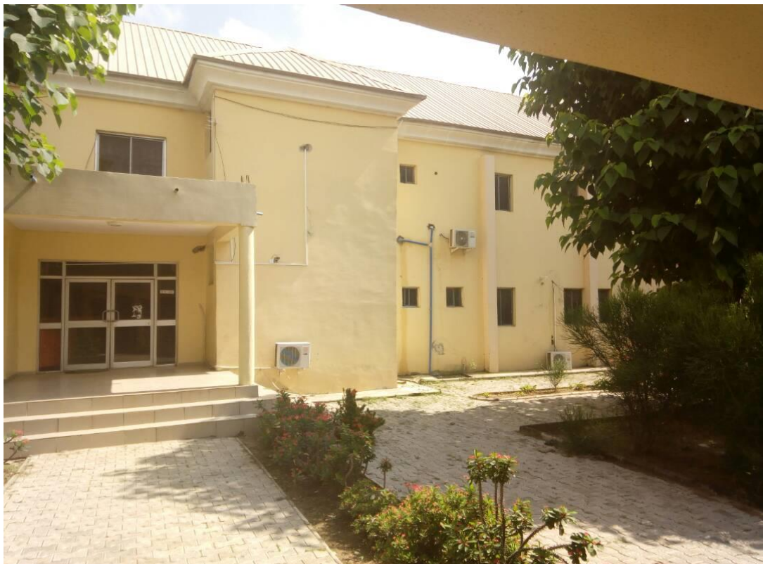
Figure 15. Front View of FOMWAN Hostels at Its National Headquarters, Abuja
