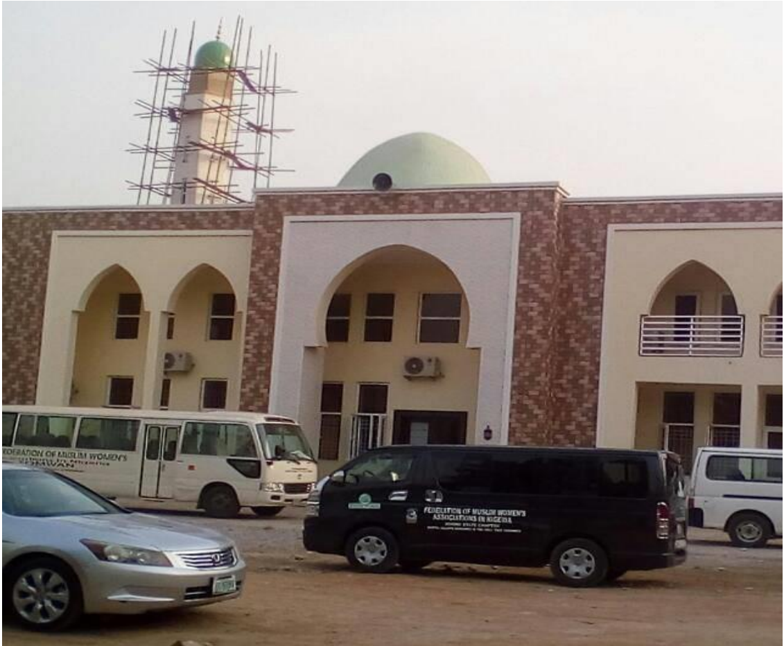
Figure 14. FOMWAN Central Mosque, National Secretariat, Abuja
