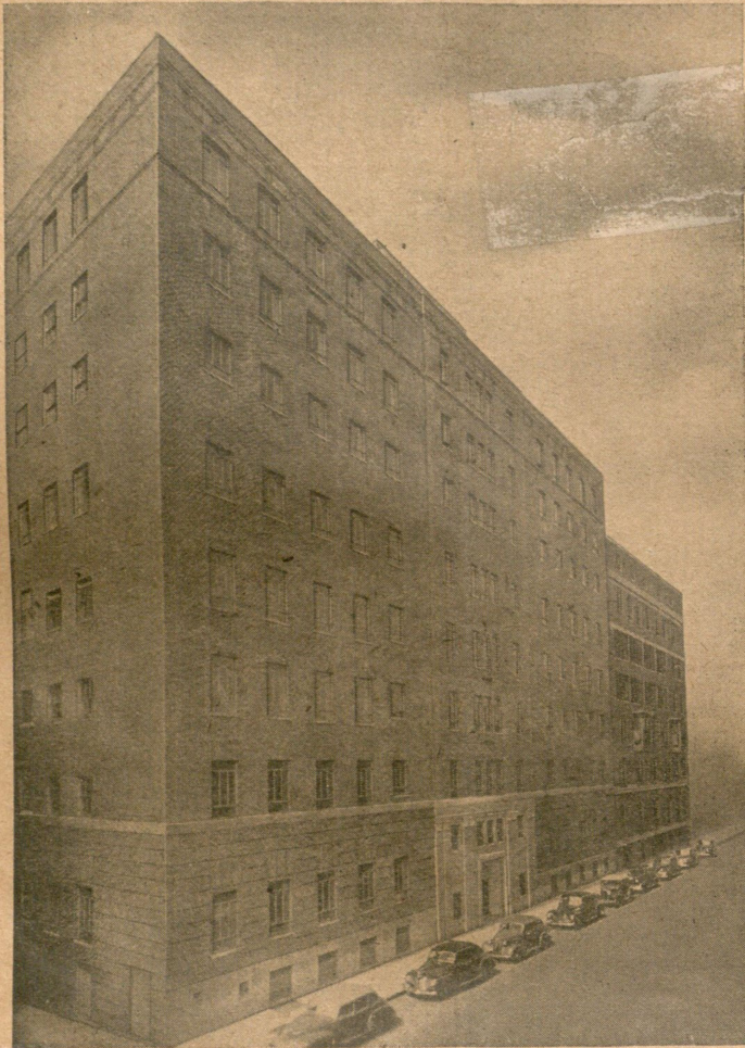
Newton Street View of the New Evans Memorial Hospital
