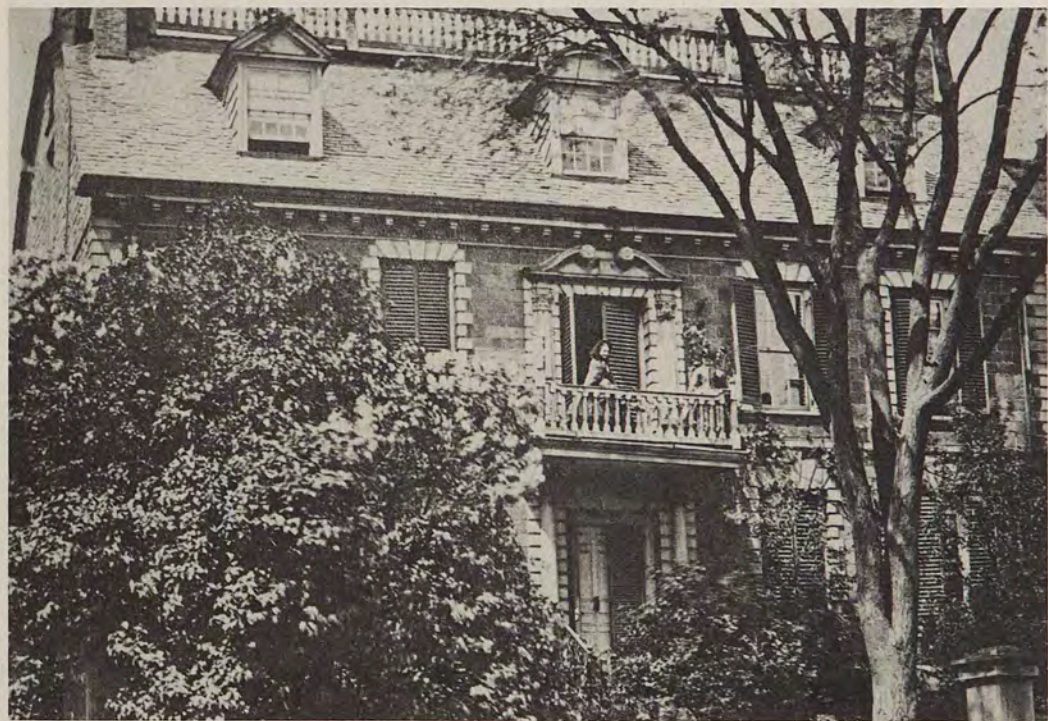
Figure 4 Balcony doorway, Thomas Hancock house, Boston, 1738-1740. (photographed ca. 1859-1863)
