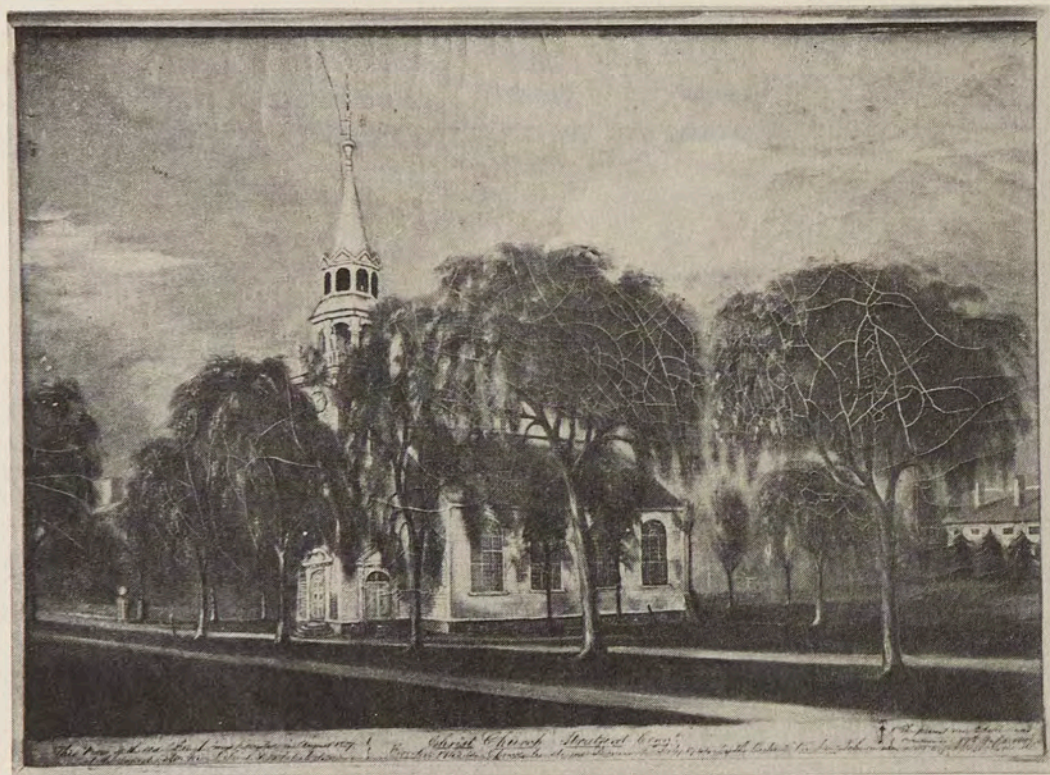
Figure 7 Christ Church, Stratford, Connecticut, begun 1743, demolished 1858. From a painting dated August 1857. Christ Church, Stratford.
