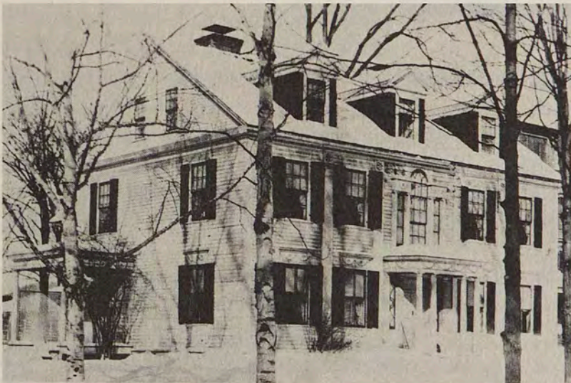
Figure 5 Perez Jones house, Windsor, Vermont, 1800-1801. Designed and built by Asher Benjamin. (photograph ca. 1945)
