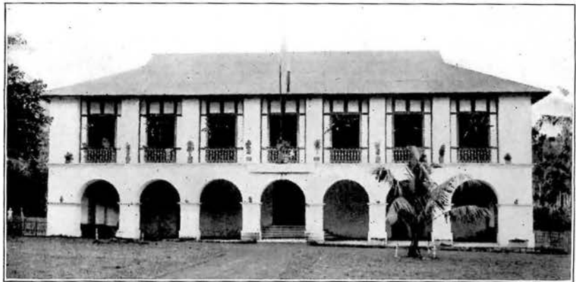
Libog Central School building, Libog, Albay, reconstructed out of roofless and floorless tribunal dating from the Spanish régime.
