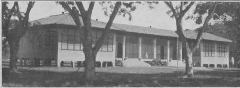
Butuan Central School building, Butuan, Agusan.
