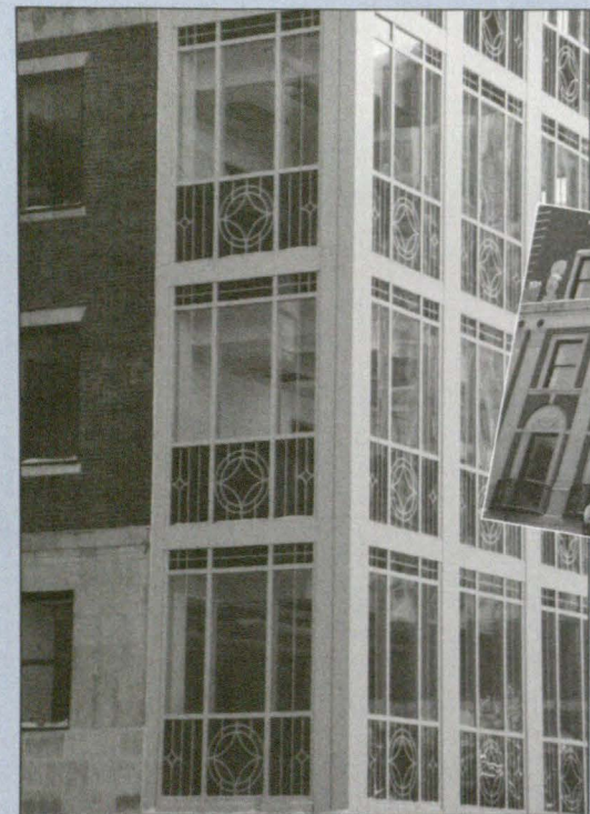
Architectural details, 85 East Concord Street
