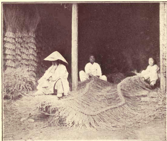
MAKING THE ROOF THATCH.
