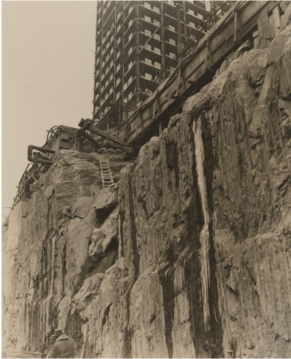
Figure 3.29. Berenice Abbott, Rockefeller Center 30 Rockefeller Center (foreground excavation), completed 1933; Radio City Music Hall (background construction), completed 1932, New York, photograph, 1931-32, Philadelphia Museum of Art, 2001-62-9.
