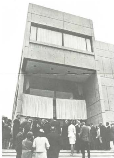
Above, Watch this space! Curtains are drawn across the simple but impressive facade of the new School of Graduate Dentistry on the day of its official dedication. All eyes are turned on the granite strip above the great glass windows . . . Below, Unveiling has taken place and Dean Henry Goldman and Mrs. Rubenstein beam below the name revealed: "The Lawrence J. and Ann Cable Rubenstein Building — Boston University School of Graduate Dentistry."
