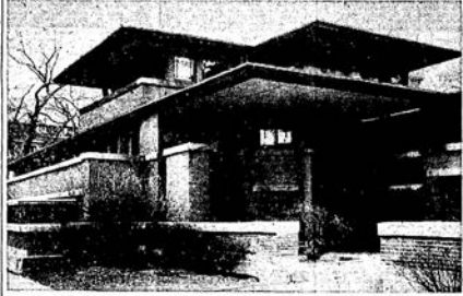
Robie house at 5747 Woodlawn av. designed more than 50 years ago by Frank Lloyd Wright, which the owner, Chicago Theological seminary, wants to replace with an apartment building for married students.
