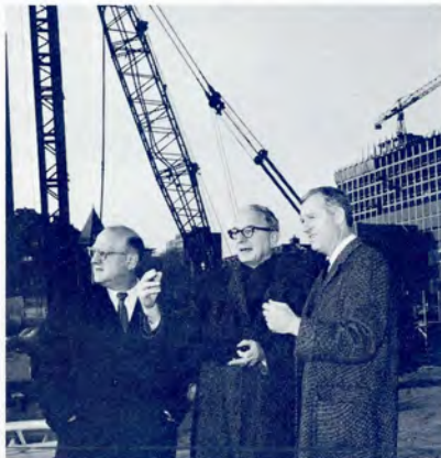
5. Checking the site for the School of Graduate Dentistry building were (left to right) the School's Dean Henry M. Goldman, Medical Center Director Lewis H. Rohrbaugh, and University President Arland F. Christ-Janer. Dedication ceremonies for the 4-story structure will be held on September 7-9, 1969.
