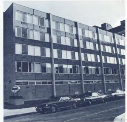
At left, the Doctors' Office Building and garage, for Center physicians. Above, the 160-bed Medcenter, extended care facility.
