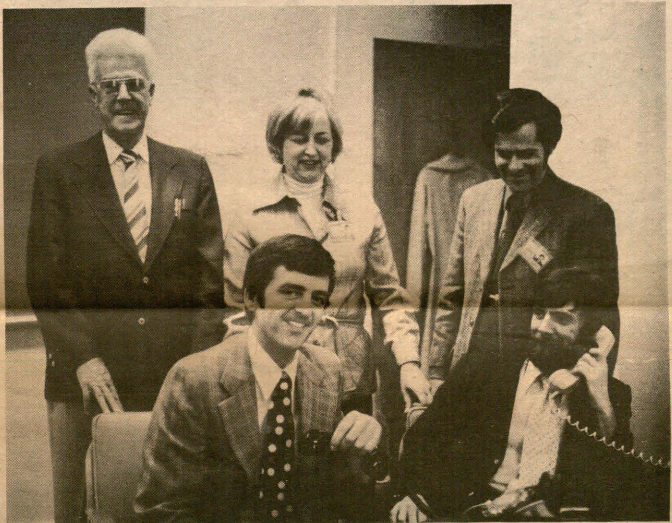
THE SWITCHBOARD - The switchover to Centrex was planned and directed by the Centrex Conversion Committee. Members are, from left to right, front row, Gerald Borgal, UH general administrator for Inpatient Care Services, which includes Telecommunications; and Peter Landry, senior management engineer at UH. Pictured in the back row are, left, James Crowley, director of the mailroom at the Medical Center; Patricia Tobin, assistant to the director for Telecommunications at UH; and Edwin Stedman, director of Security and Telecommunications, UH.
