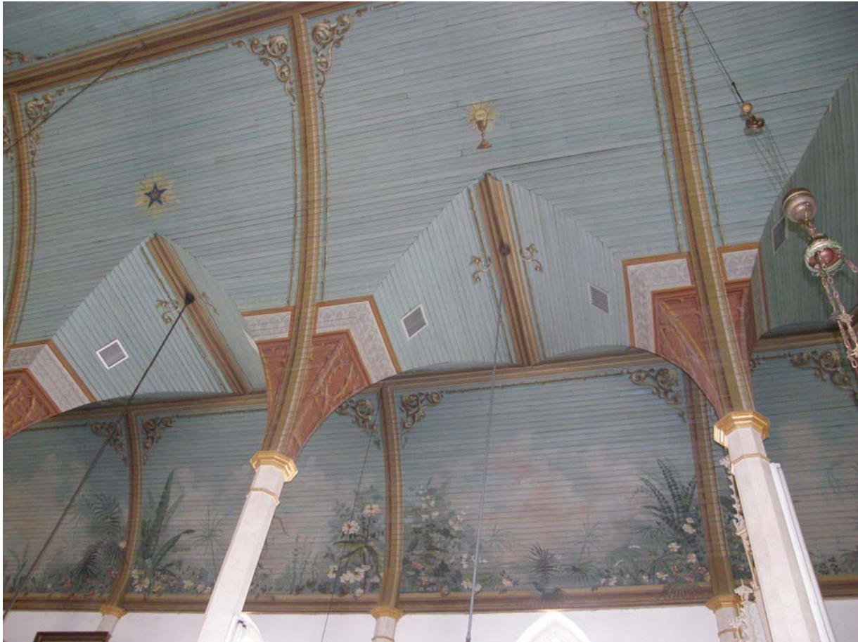
Figure B9. Ceiling of St. Mary's, Praha, TX
