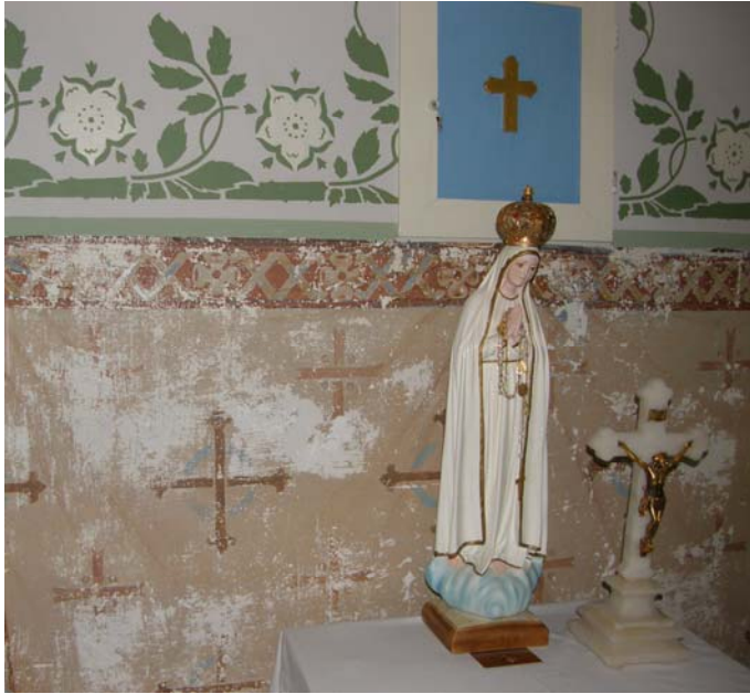
Figure B7. Original paint revealed during restoration
