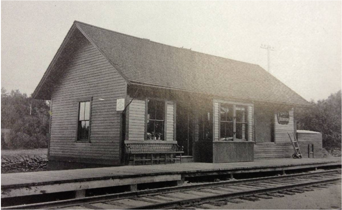
Fig. 50: At East Hebron, an inherited combination station, the directors of the Portland & Rumford Falls Railway eventually added a projecting window for the station agent. Notably, it carried the varied exterior patterning like other stations designed by Lewis & Danforth, but not the rest of its own exterior. [Lewis, New England Country Depots ]
