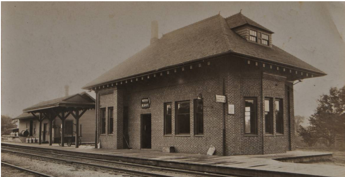
Fig. 51: When West Minot outgrew its combination station, built in the 1870s (left), it added a dedicated brick passenger station (1899) as was common of railroads who had moved beyond initial development and could command greater funds for station construction. [Courtesy MHPC]
