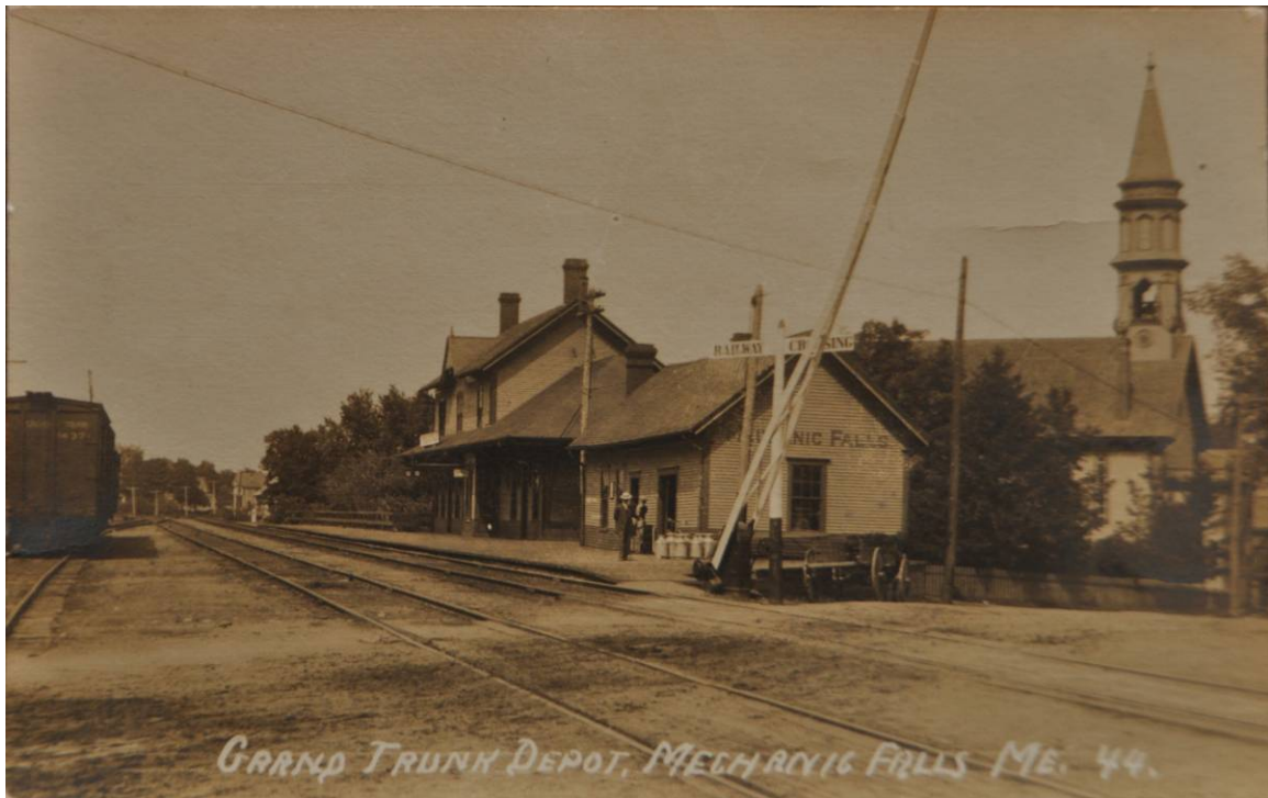
Fig. 58: In replacing an inherited station at Mechanic Falls (Fig. 31), the Portland & Rumford Falls Railway sought to upstage the existing station of its competitor, the Grand Trunk Railway, at Mechanic Falls. The Grand Trunk's two-story passenger depot is in the background and its freight depot in the foreground. Across the tracks (not pictured) were the Portland & Rumford Falls Railway's buildings (see Fig. 59). [Courtesy MHPC]
