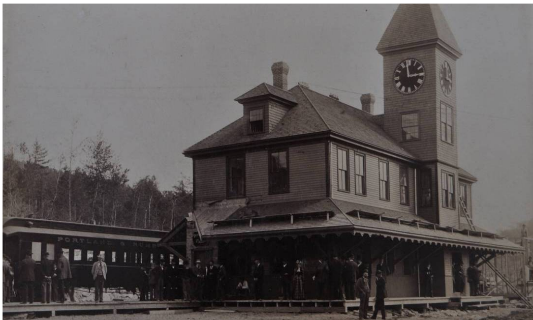
Fig. 12: Rumford Falls Station under construction, 1893. [Courtesy MHPC]
