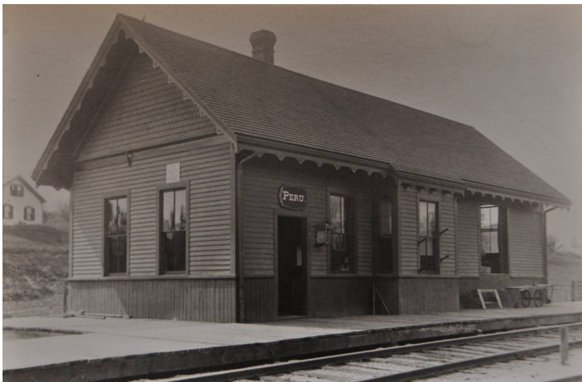
Fig. 21: Peru, a new station, was one of Lewis and Danforth's standard combination depot designs on Extension A. [Courtesy MHPC]
