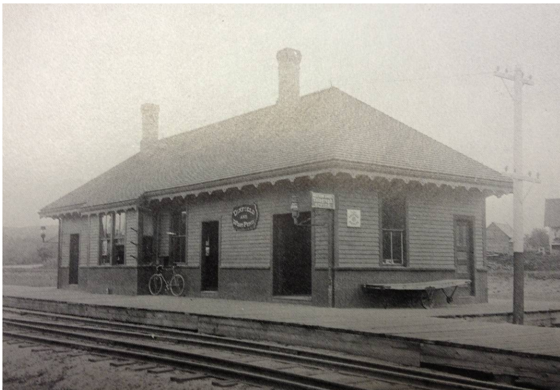
Fig. 17: Dixfield/West Peru Station, built 1892. Note that the building as constructed was “flipped” from the floor plan (Fig. 18). [Lewis, New England Country Depots ]
