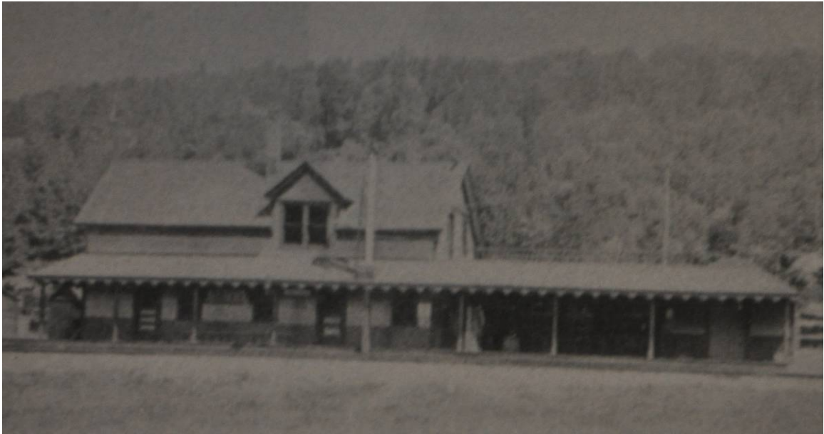
Fig. 42: Roxbury passenger station (1895) on the Rumford Falls & Rangeley Lakes Railroad featured living quarters for the station agent upstairs and a separate freight depot connected by a midway. [Hutchinson, The Rumford Falls and Rangeley Lakes Railroad ]
