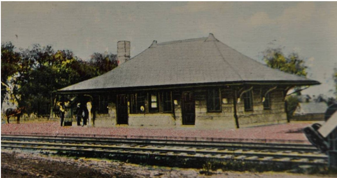
Fig. 53: Shortly before the Maine Central assumed the Portland & Rumford Falls Railway, it replaced the Mechanic Falls passenger station with a stone structure (1906). [Courtesy MHPC]
