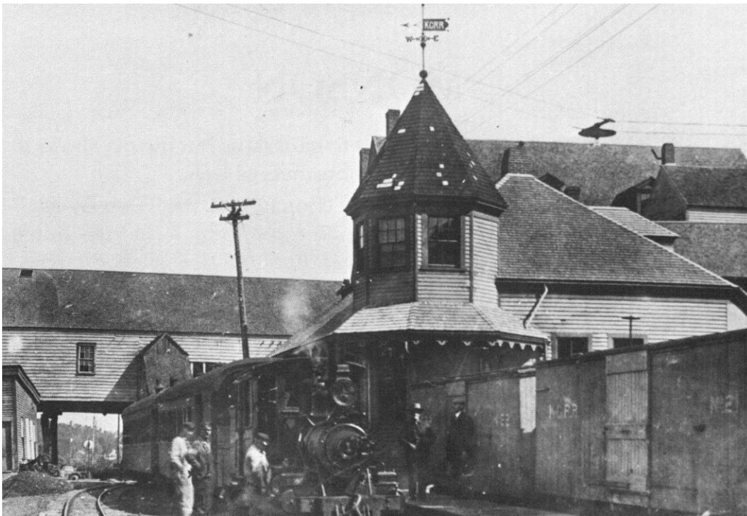
Fig. 7: Randolph Station (1890) where Lewis used Queen Anne styling, including a corner turret and decorated bargeboards. [Courtesy MHPC]
