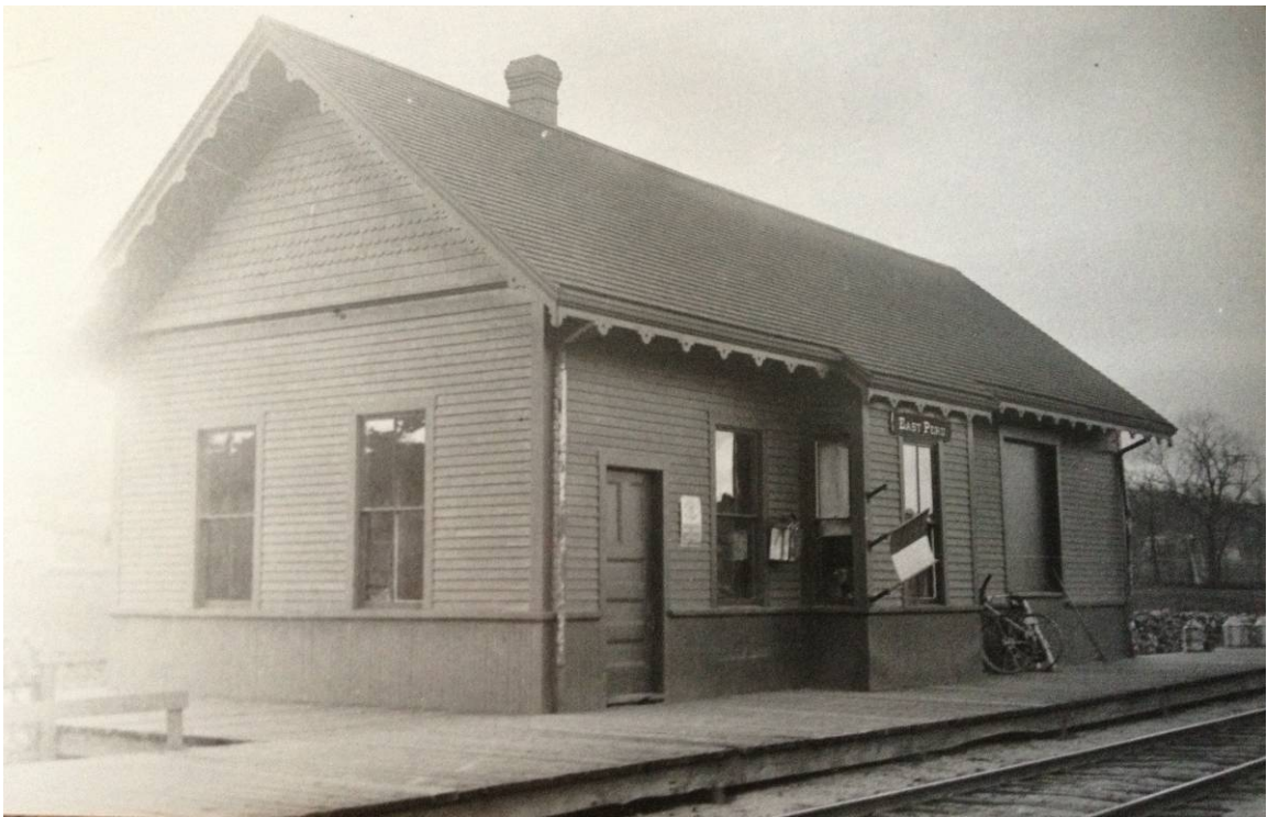
Fig. 20: East Peru, a new station, was one of Lewis and Danforth's standard combination depot designs on Extension A. [Courtesy MHPC]
