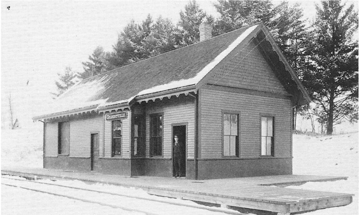
Fig. 19: Gilbertville, replacing an existing station, was one of Lewis and Danforth's standard combination depot designs on Extension A. [Lord, Downeast Depots ]
