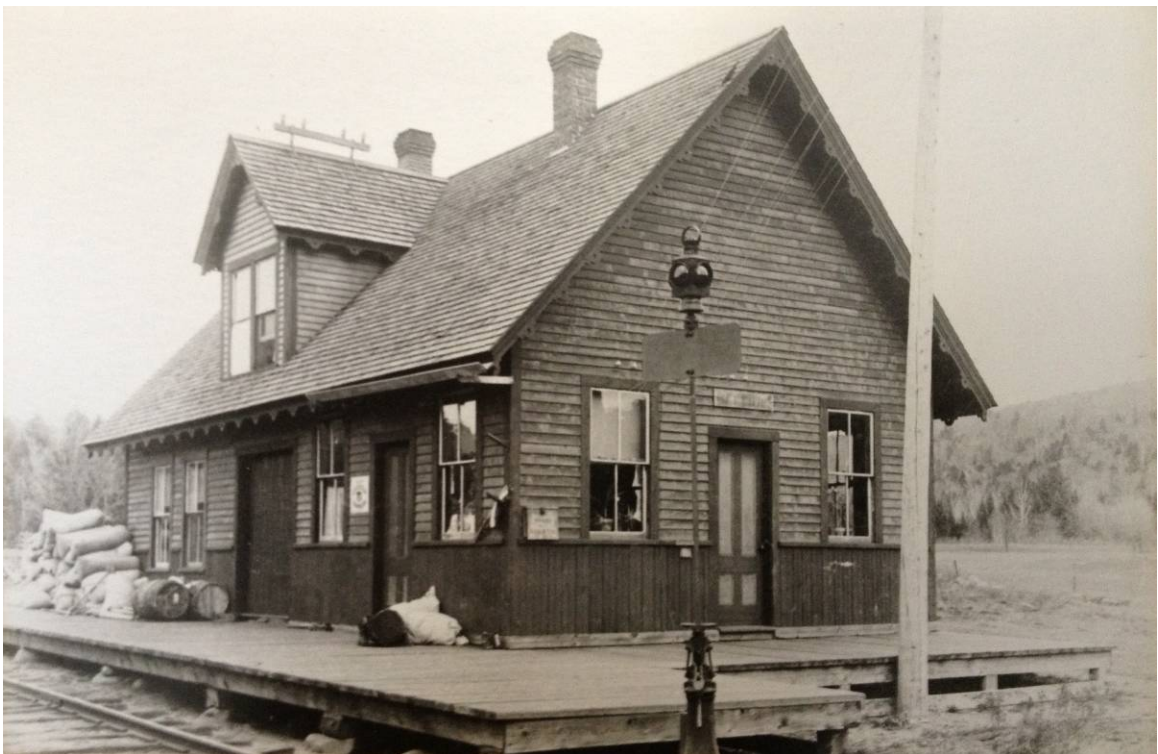
Fig. 41: An unusual configuration of combination depot at Houghton contained living space for the station agent, but continued the design schema of the other stations on the Rumford Falls & Rangeley Lakes Railroad. [Courtesy MHPC]
