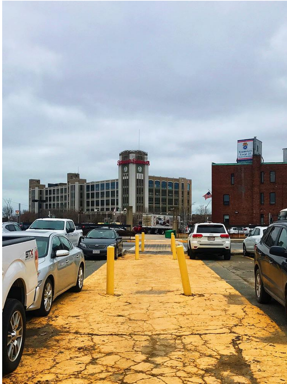
Figure 6: A view of the refurbished chocolate factory which houses the Coalition, along with many other businesses (Bailey 2018)
